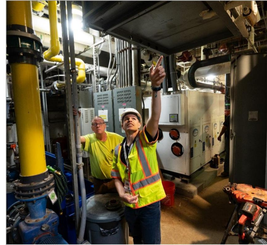
Reston Community Center Heating System Upgrade
